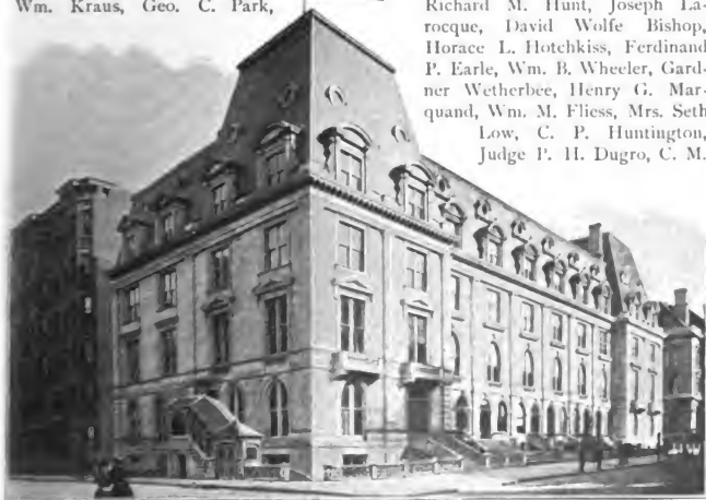
PLAZA BANK, FIFTH AVENUE, SOUTHEAST CORNER OF 58TH STREET.
